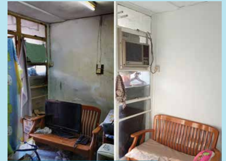
Story 3 - Comparison before and after renovation
